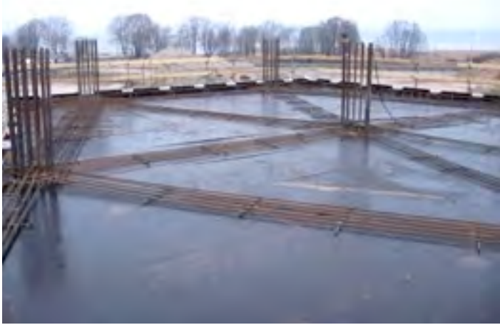
APC-reinforcement in bottom layer; top reinforcement at cantilevers and statically determined areas
