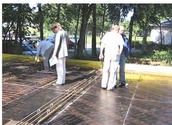
installation of APC-reinforcement in bottom layer on the day of casting concrete; in areas of statically determined structures a combination of sfrc and traditional reinforcement is regarded (here: top reinforcement d=8mm, e=150mm at cantilever)
