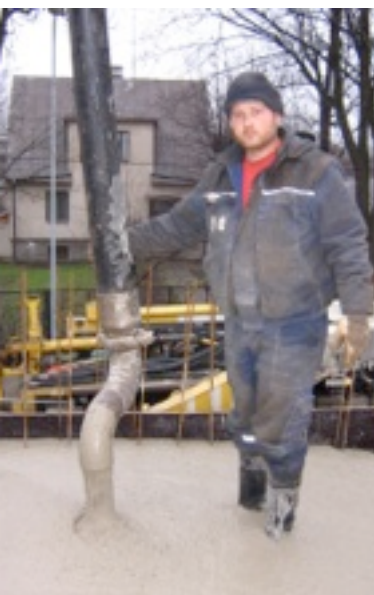
easy pumpability due to adapted concrete design as almost self compacting concrete; clean and smooth results
