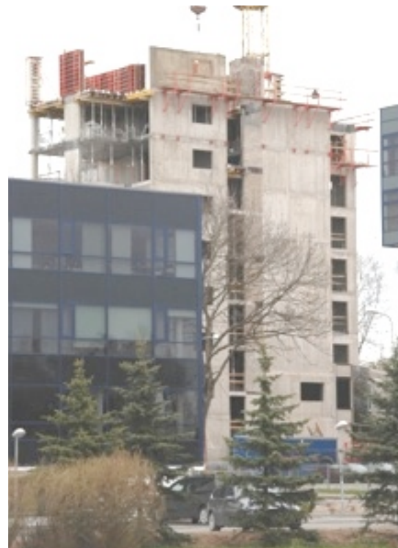
fast installation: except some Anti-Progressive-Collapse-Reinforcement in the bottom layer no additional reinforcement installed. APC-rebars were installed on the day of pouring in the morning
