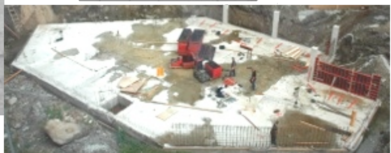
foundation floor d=800mm; sfrc pumpable with standard concrete pumps and rubber pipes.
