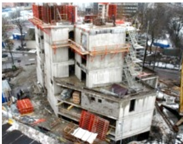
fast installation: except some Anti-Progressive-Collapse-Reinforcement in the bottom layer no additional reinforcement installed. APC-rebars were installed on the day of pouring in the morning
