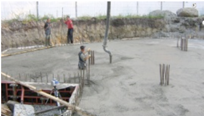
foundation floor d=800mm; sfrc pumpable with standard concrete pumps and rubber pipes.
