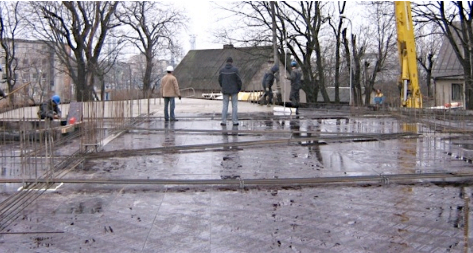
fast installation: except some Anti-Progressive-Collapse-Reinforcement in the bottom layer no additional reinforcement installed. APC-rebars were installed on the day of pouring in the morning
