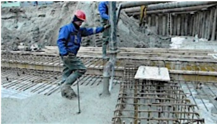
fast installation process (1 field per day including all additional reinforcement)
