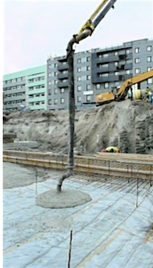
easy pumpability and workability; Severstal-metiz concrete design in cooperation with the concrete supplier
