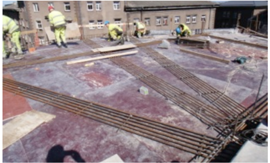
installation of APC-reinforcement in bottom layer on the day of casting concrete
