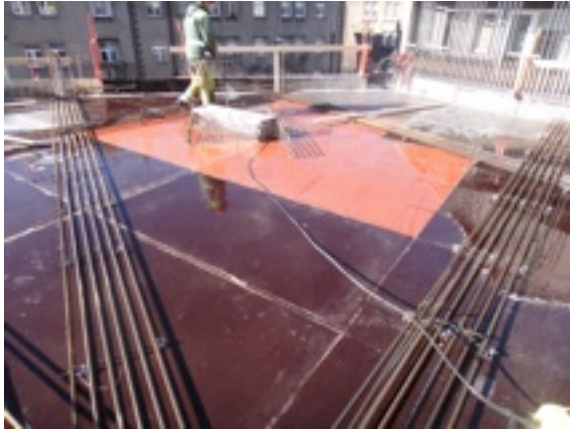
installation of APC-reinforcement in bottom layer on the day of casting concrete
