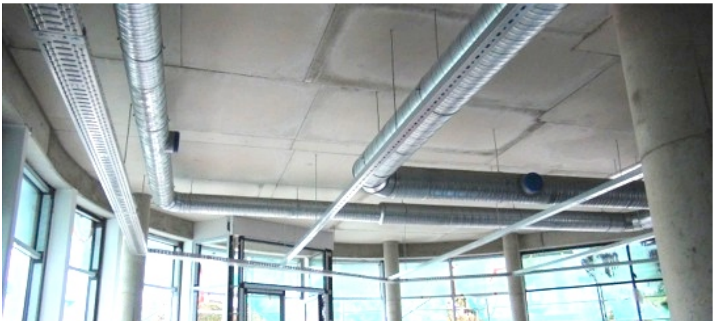
bottom surface with ultra fine texture due to low viscosity of almost self compacting concrete
